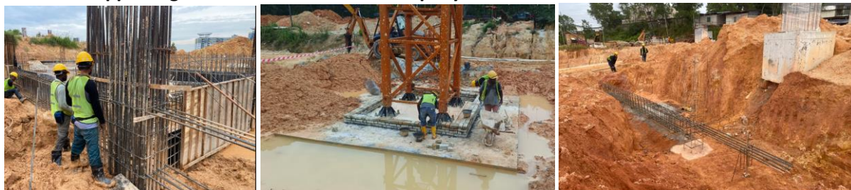
Frame panel formwork installation and civil engineering
